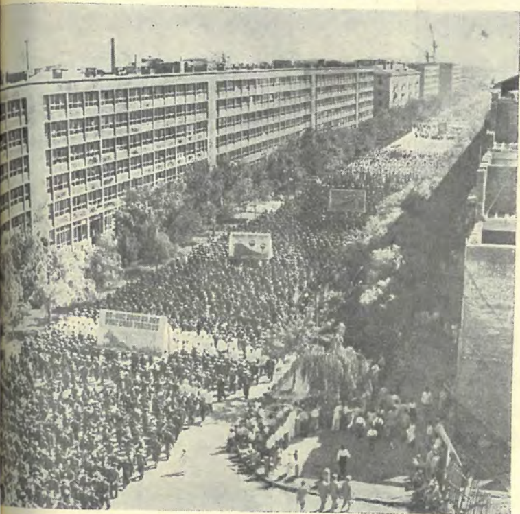
Ranks of socialist builders marching through the street lined with grand new buildings
