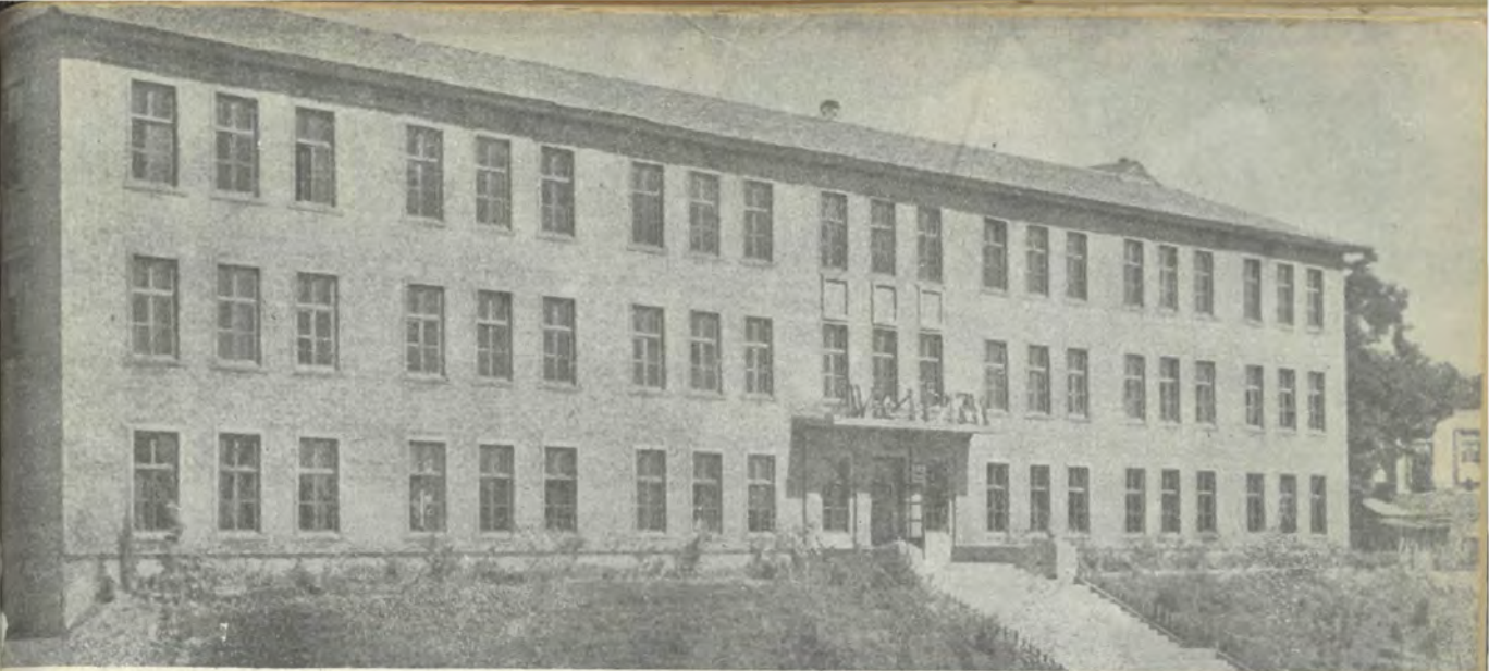
A view of the building of the Pyongyang Middle School No. 8
