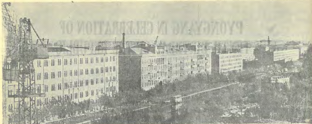
A part of Pyongyang city under construction
