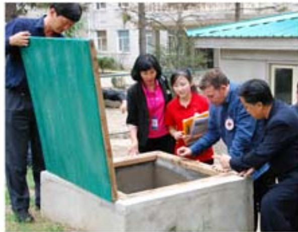
A water supply and sewage project has finished in cooperation with the International Federation of the Red Cross and Red Crescent.
