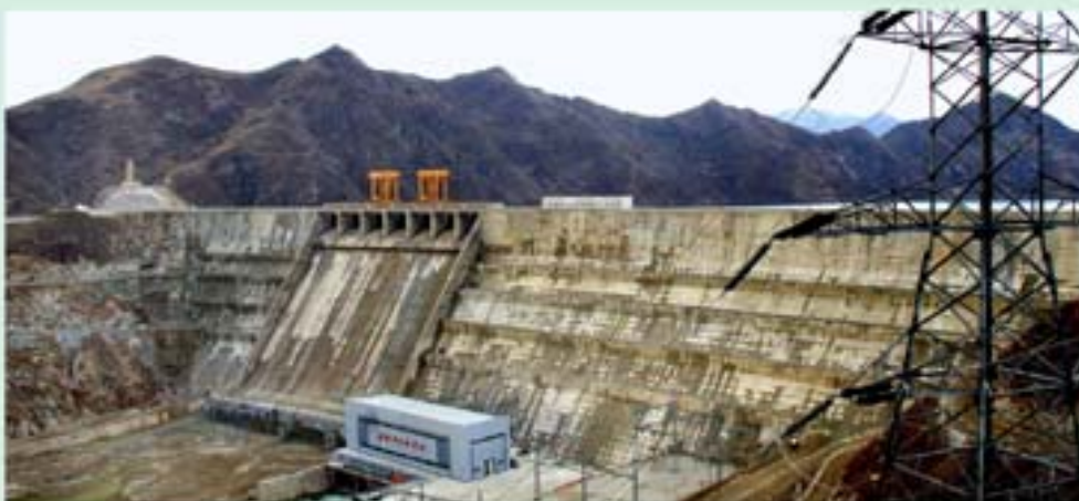
Plant No. 2 of the Huichon Power Station built by People's Army soldiers.
