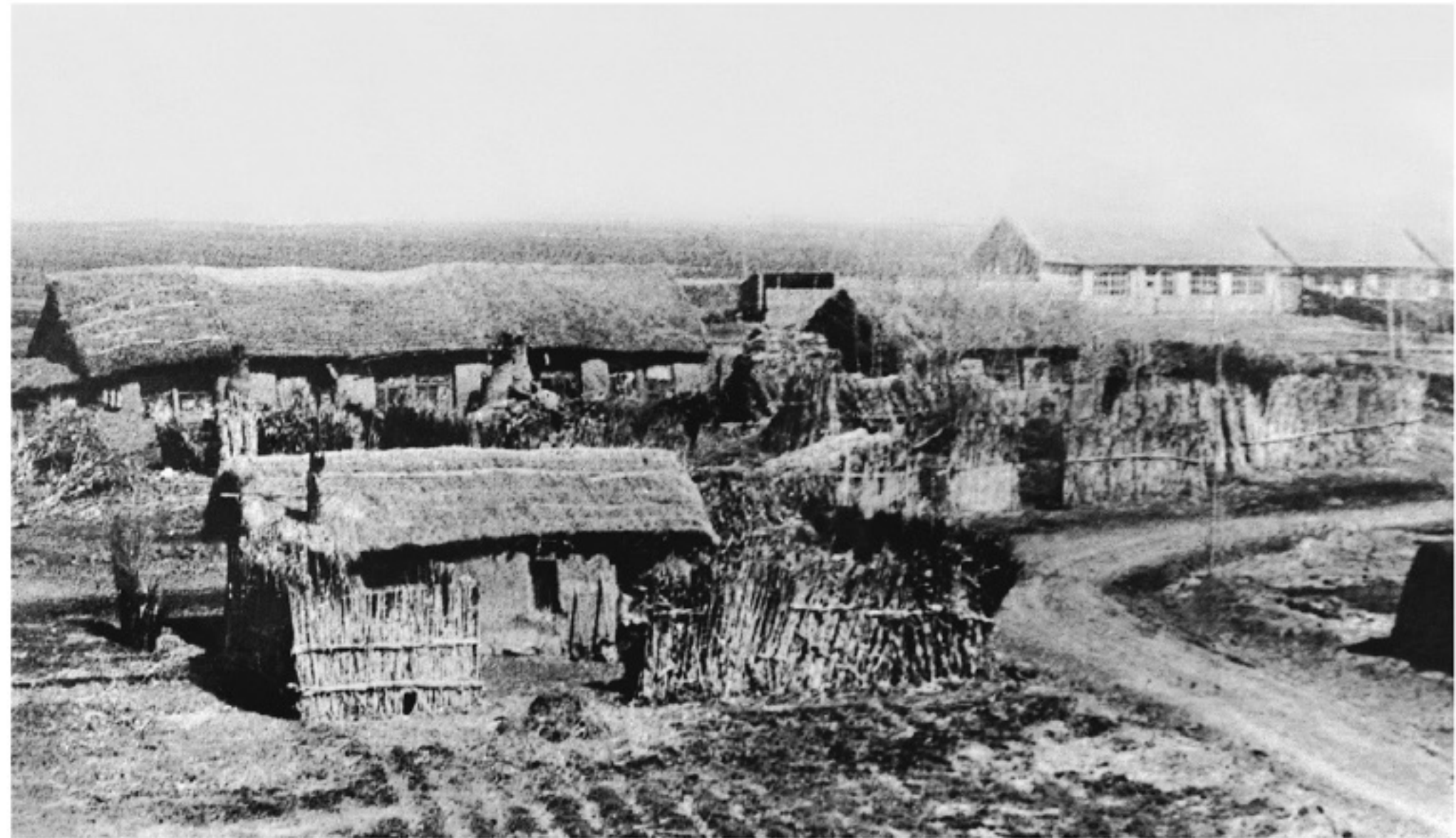
Jiajiatun village where the historic Kalun meeting was held and the first party organization was formed
