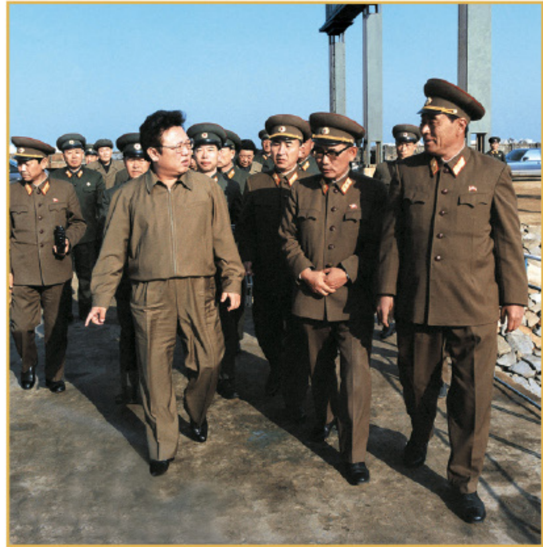
Kim Jong Il giving field guidance at the construction site of the West Sea Barrage (April 1984)
